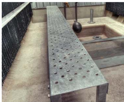
Internal Maintenance Walkway:
