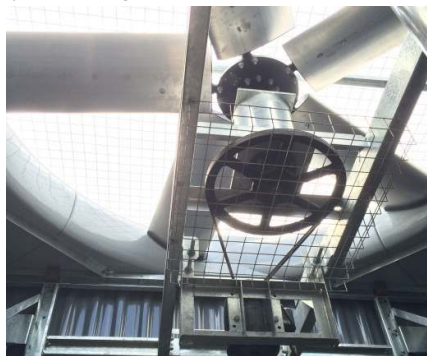
Driven system inside CT: Maximize reduce static & Delivery more airflow
