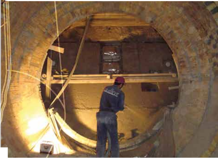
Installation of Refractory Material by "Gunning"
