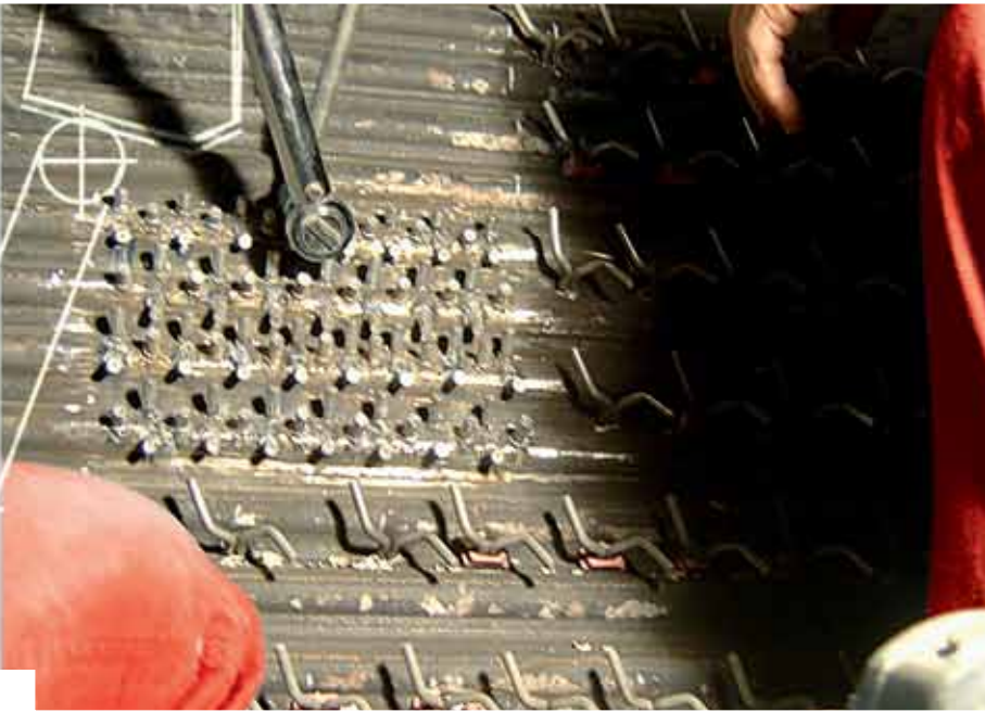
Welding of special MVP anchors and studs
