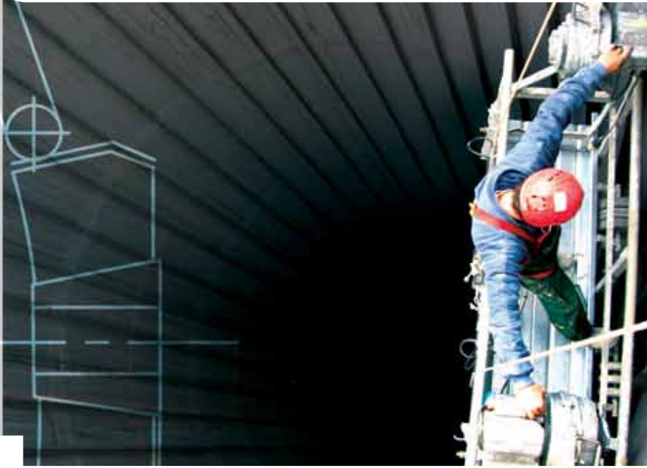
Inspection of metal chimney (inner part)
